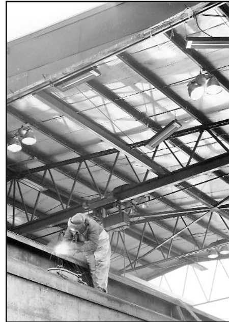
Photo 4-8: Welder at Work. Electric IR units mounted below building ceiling provide comfort heating. Photograph compliments of Fostoria Industries, Inc.
